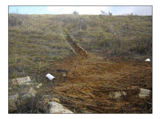
Plate 7 Lower: Possible seepage from the northern KVAR embankment, above Site 3, following a large rain event.
