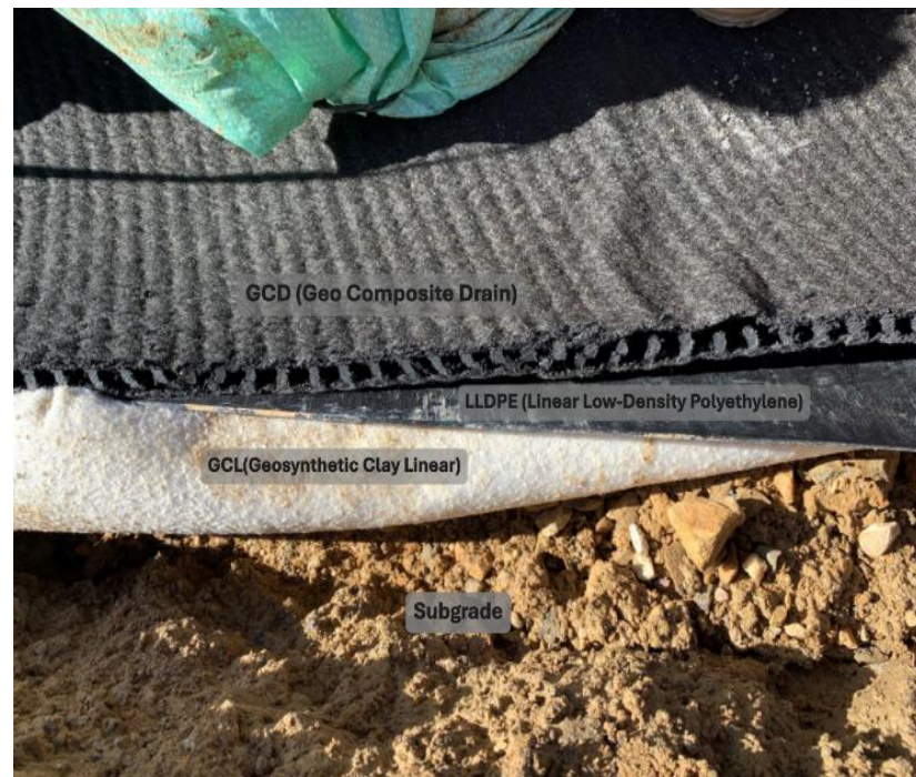
Photo 5: Engineered Leachate Barrier Management System showing the multiple layers in its design (February 2024)
