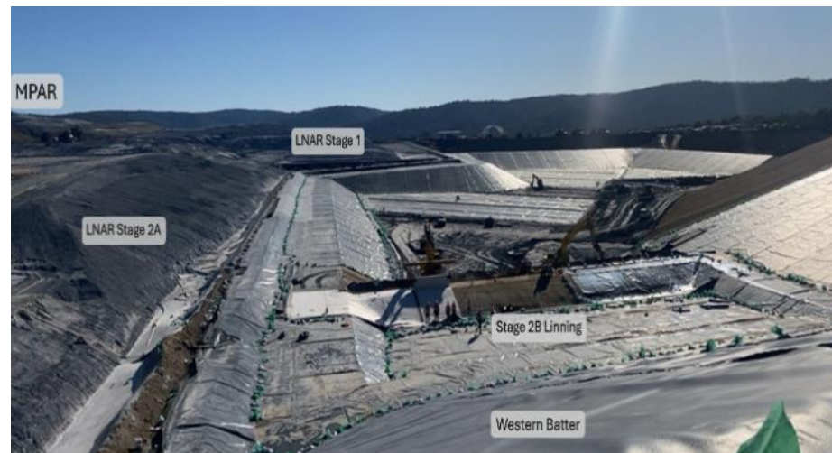
Photo 3: Installation of Liner at LNAR Stage 2B (April 2025)
