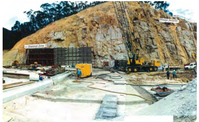
Lake Lyell Spillway Widening c. 1994
