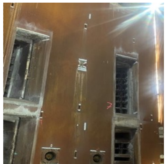
Burners Refurbished
