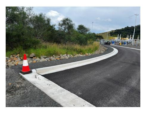
Photo 3: GPRS area sealed with permanent drainage in place
