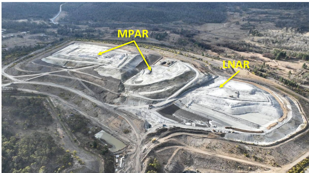
Plate 2 Aerial view of Mount Piper Ash Repository (MPAR) and LNAR Stage 1 (A and B) areas (Photo taken 16 August 2023)
