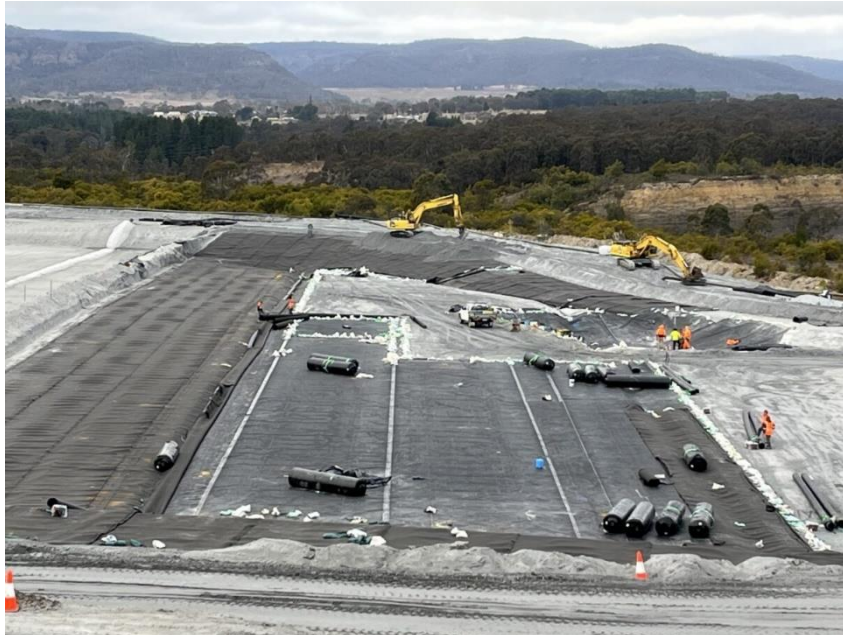
Plate 3 Installation of the liner at LNAR Stage 1B (Photo taken 24 July 2023)
