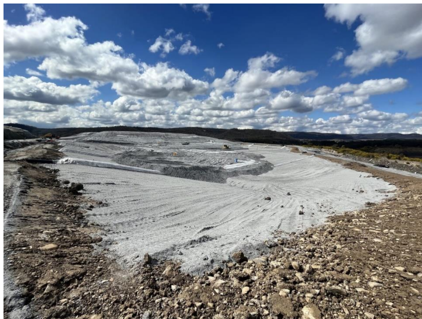
Plate 4 Ash Placement in LNAR Stage 1B (Photo taken 17 August 2023)
