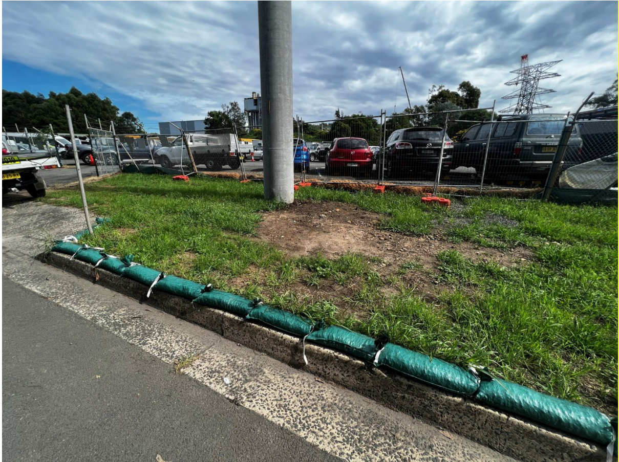
Photo 9: Sediment control in place adjacent to work area
