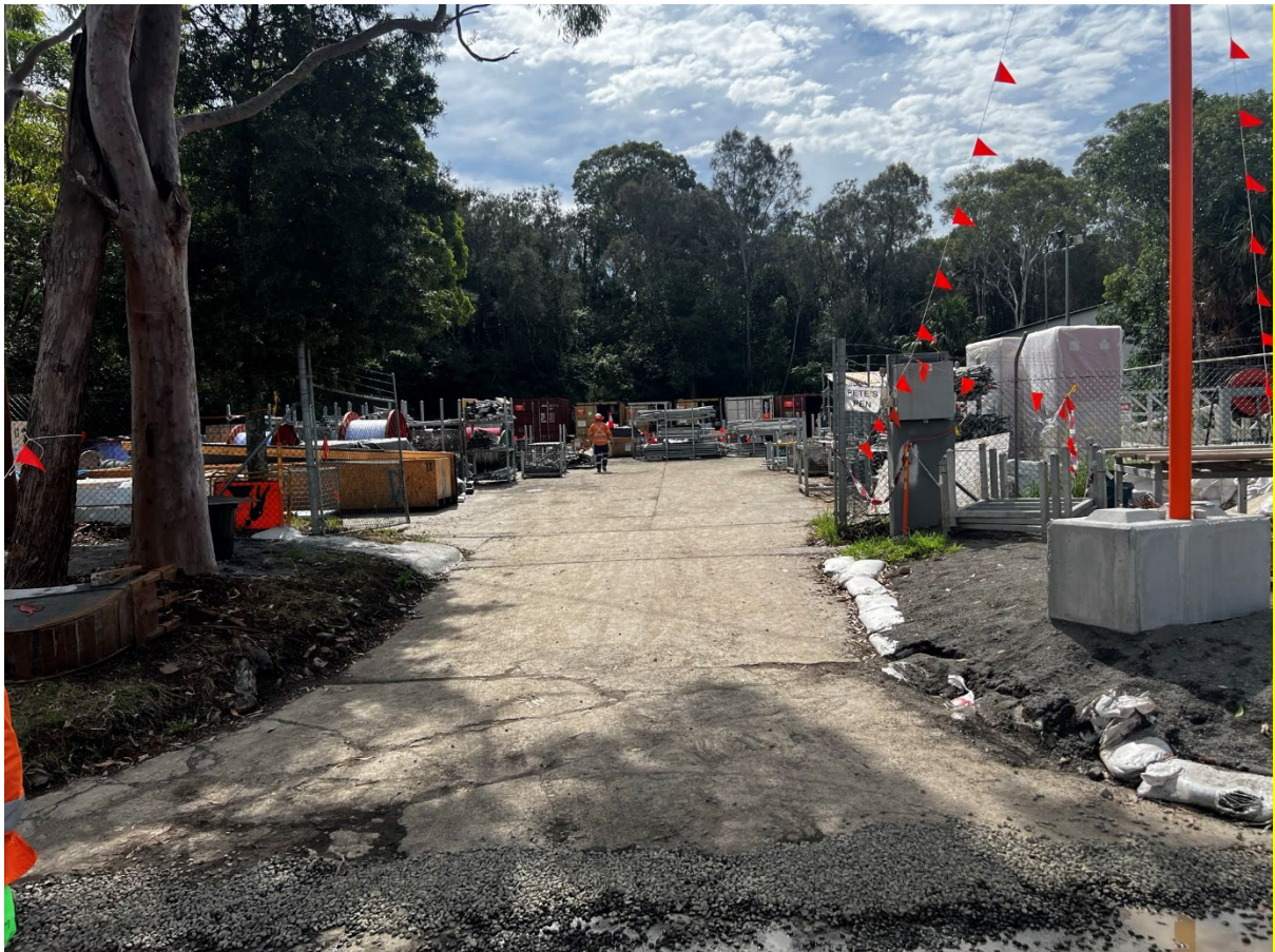
Photo 4: Ground stabilised in material storage area
