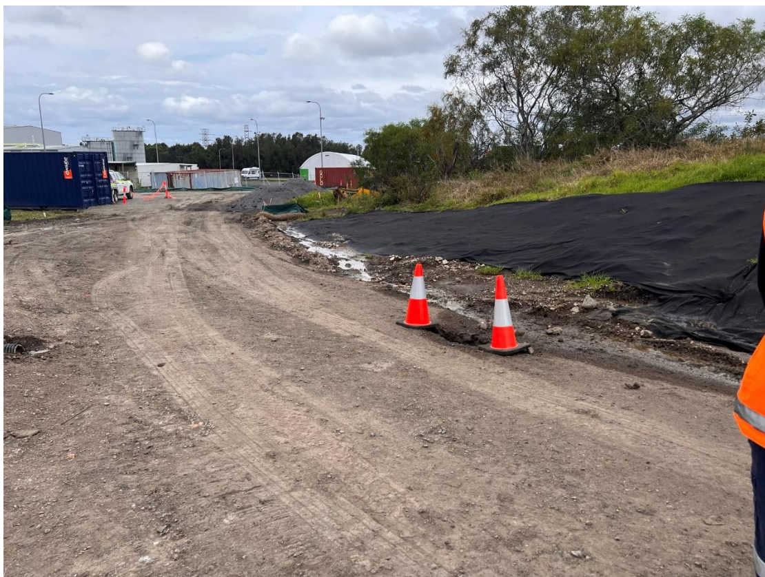
Photo 2: Erosion & sediment controls are in place and drainage is being repaired & adapted to redirect water away.
