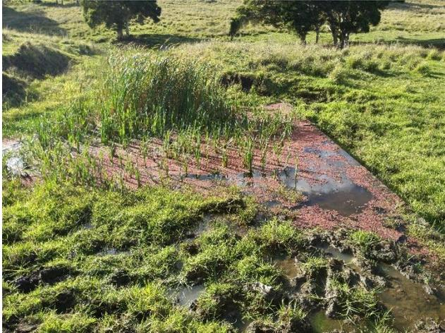
Figure 3-2 Bio-retention pond within drainage line
