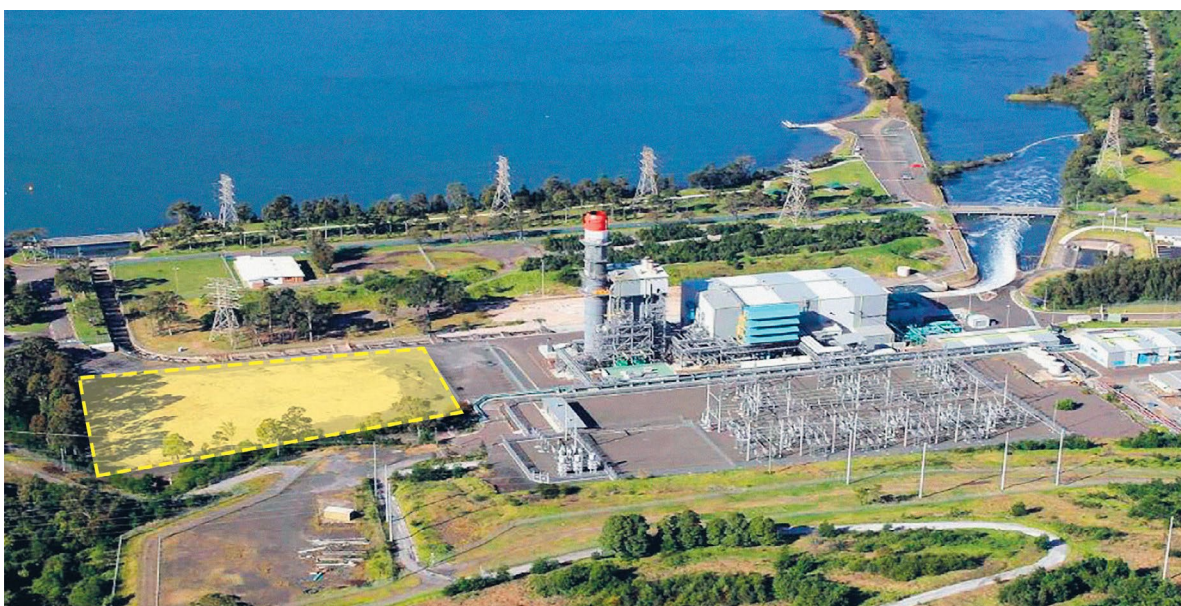
Above: EnergyAustralia's existing Tallawarra power station. Shaded area indicative of the Tallawarra B project location.
