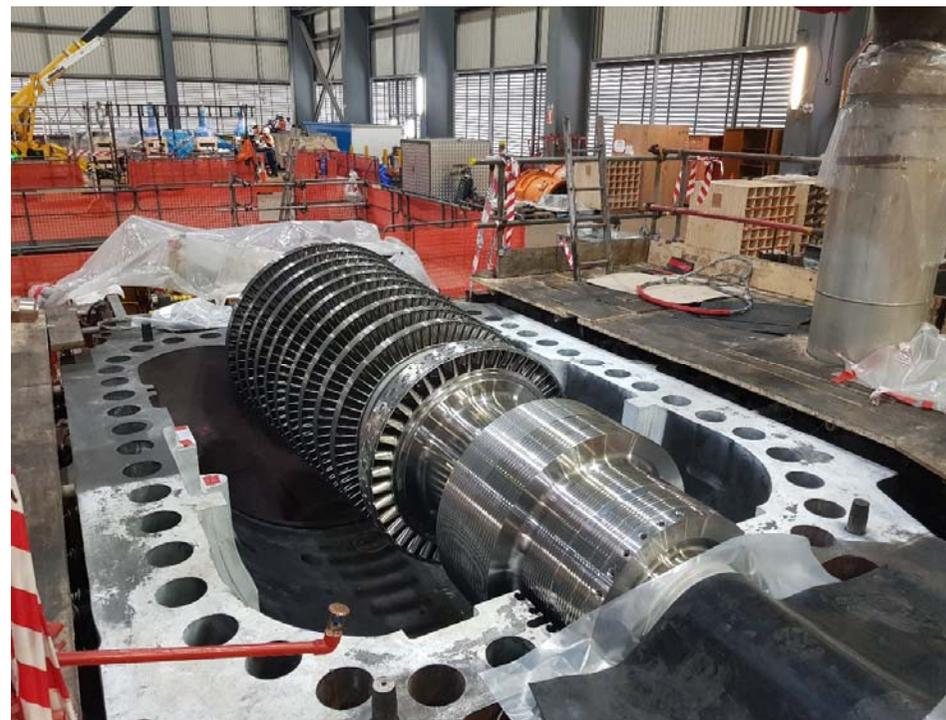
Test fitting the new High Pressure Turbine in its casing
