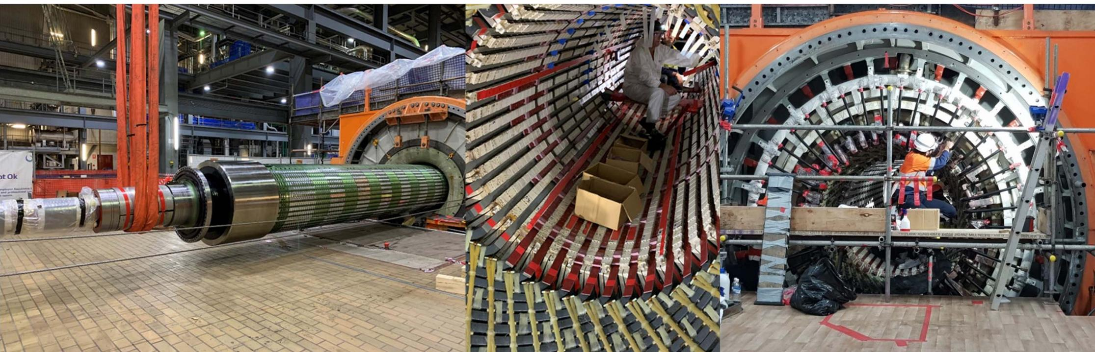
Inserting the rotor back into the generator
