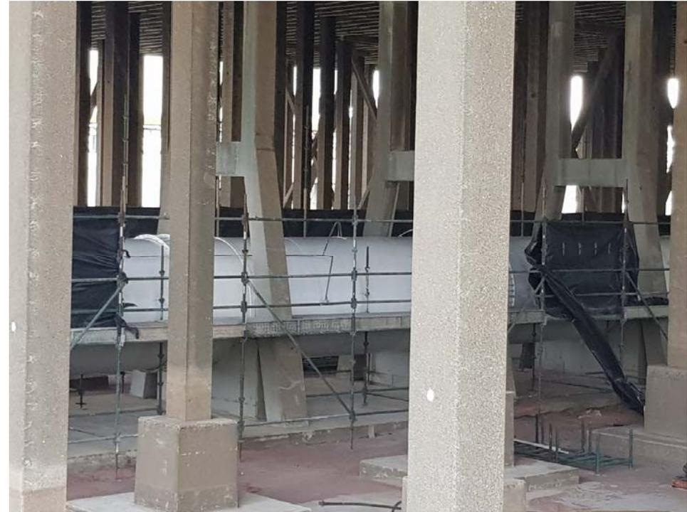
Conduit repairs in the Cooling Tower
