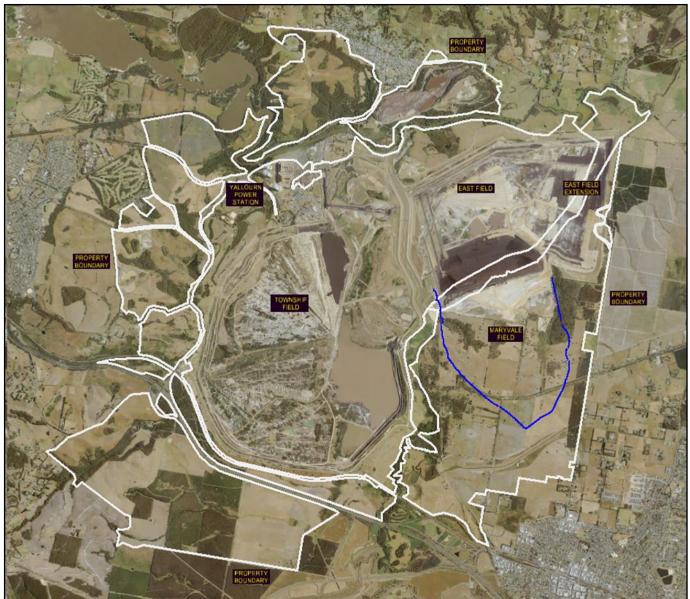
Figure 1: EnergyAustralia Yallourn Boundary - Identified in White Outline
