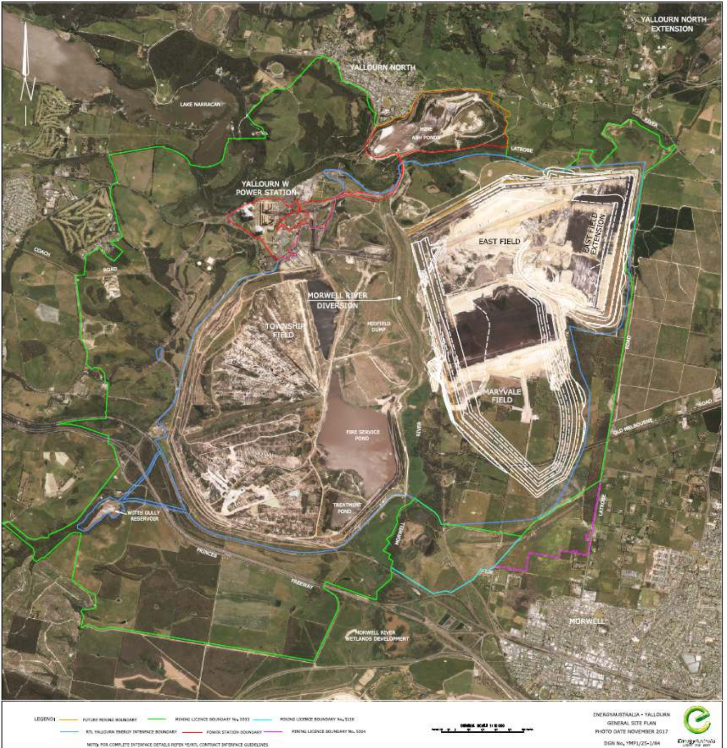
Figure 1 - Aerial Photograph of the EnergyAustralia Yallourn Site - Property Boundary Highlighted in Green
