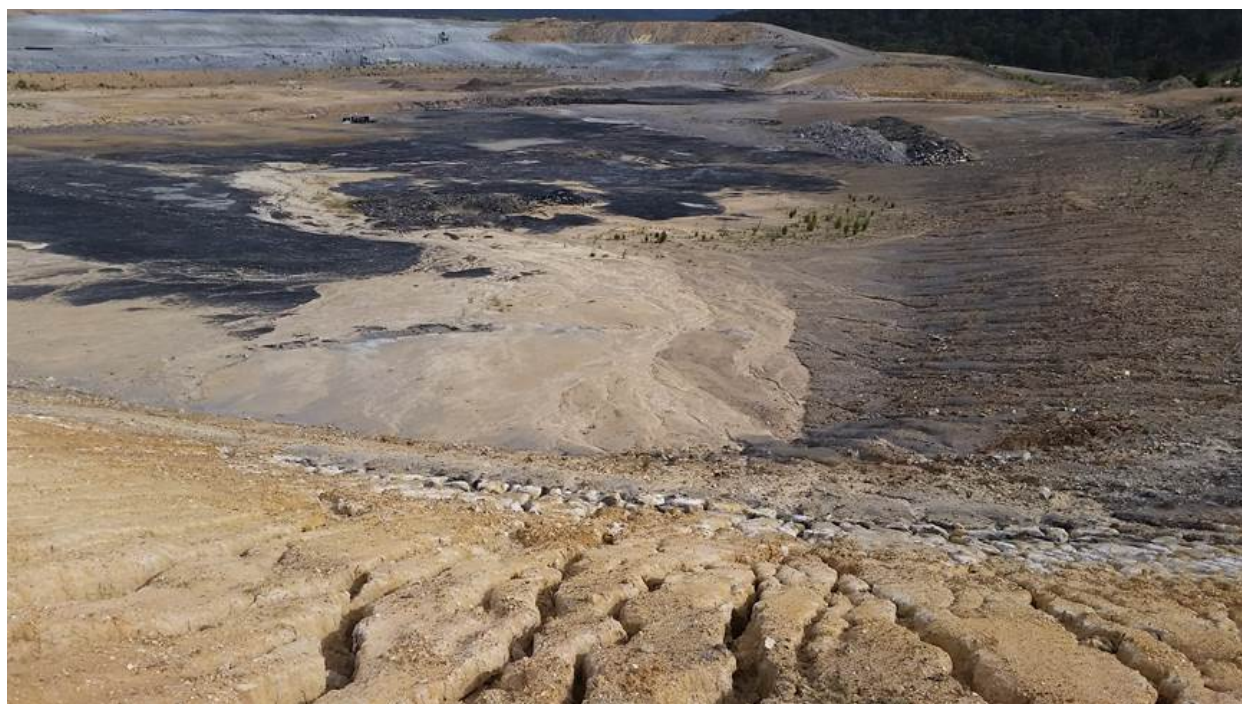
Plate 3: Excavated area of KVAR Stage 2B, containing 7.2 ha of exposed soil and coal, that requires a soil profile reinstated.
