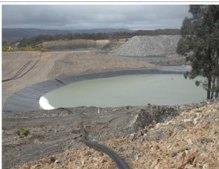
Plate 8: Lined pond collecting surface water runoff from Lamberts North
