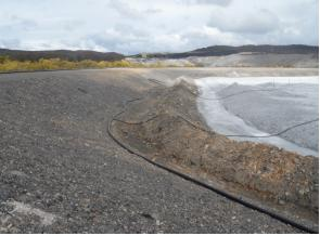
Plate 10: Drainage channels at the northern end of **Lamberts North ash placement**
