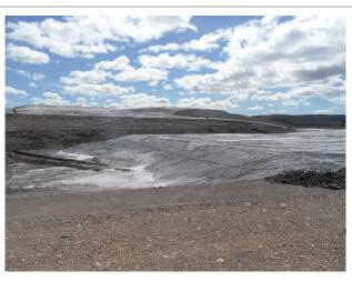
Plate 12: Ash batters with irrigation system and drainage channel
