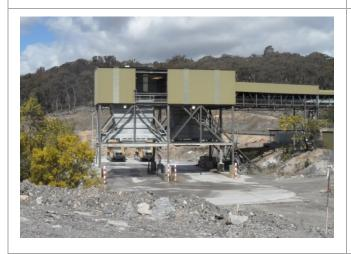
Plate 7: Ash silo near the ash placement area where ash is transferred to ash haul trucks
