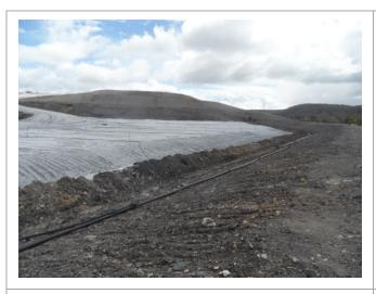
Plate 11: Drainage channels at the northern end of **Lamberts North ash placement**
