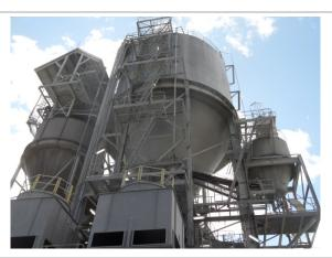
Plate 6: Ash silo at Mt Piper Power Station, prior to ash being conveyed to the ash silo near the ash placement area
