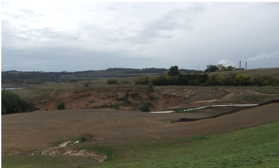
Figure 7-8: Mid Field Dump Disturbance from Morwell River Flow Toe Erosion and Circular Failure
