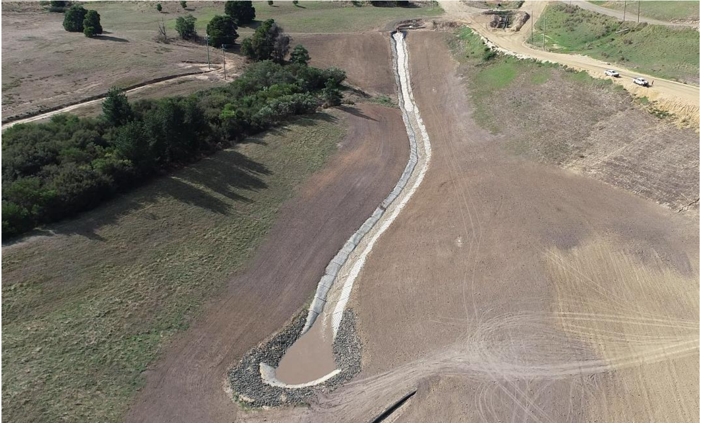
Figure 8-67: Drainage Trial Using Earthlok Concrete Mat liner, Photo Taken Shortly After Construction
