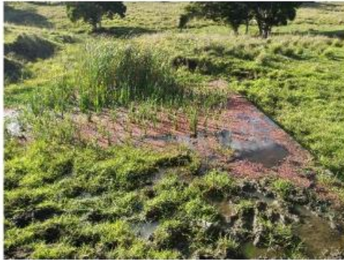
Figure 3-4 Bio-retention pond within drainage line
