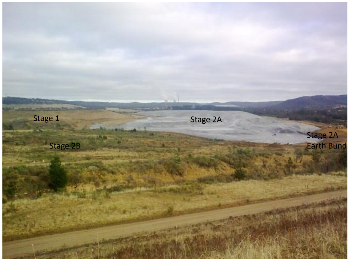
Photograph 4 View looking west back to KVAR showing Stage 1 (A & B) and Stage 2A ash placement.
