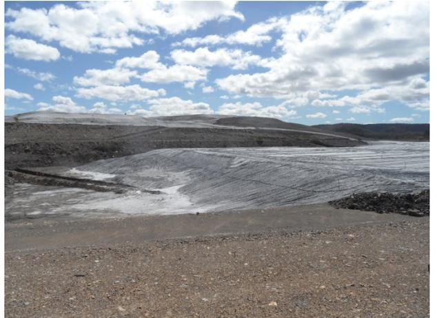
**Plate 12: Ash batters with irrigation system and drainage channel**
