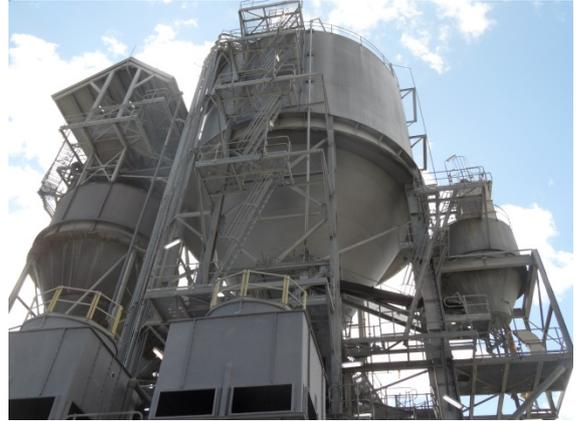
**Plate 6: Ash silo at Mt Piper Power Station, prior to ash being conveyed to the ash silo near the ash placement area**
