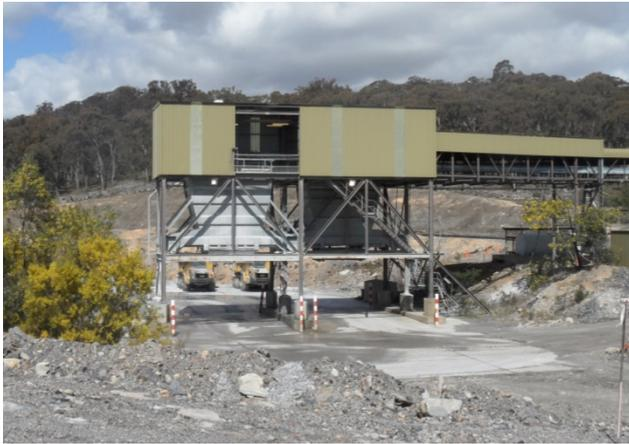
**Plate 7: Ash silo near the ash placement area where ash is transferred to ash haul trucks**
