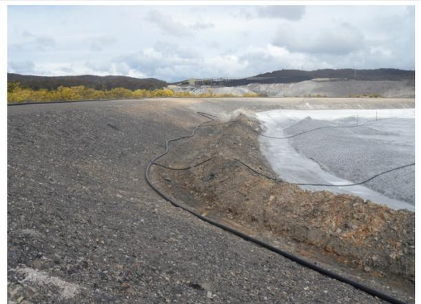
**Plate 10: Drainage channels at the northern end of Lamberts North ash placement**
