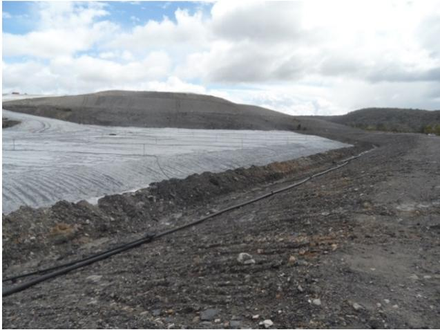
**Plate 11: Drainage channels at the northern end of Lamberts North ash placement**
