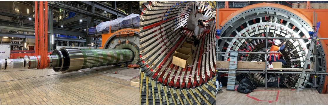
Inserting the rotor back into the generator
