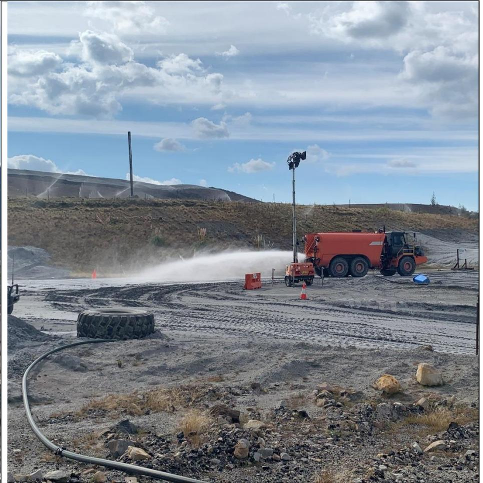
Figure 4 – Use of water cart on haul roads around Lamberts North
