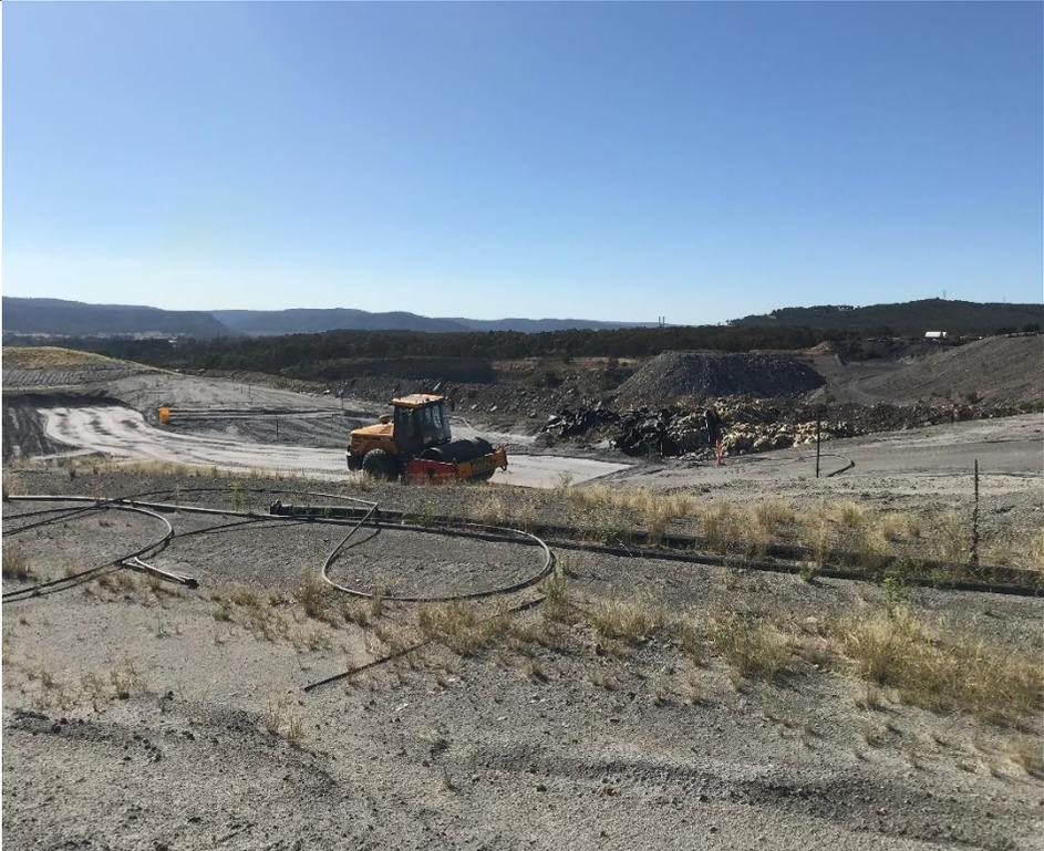
Figure 2 – Compaction activity at Lamberts North Ash Repository (January 2021)
