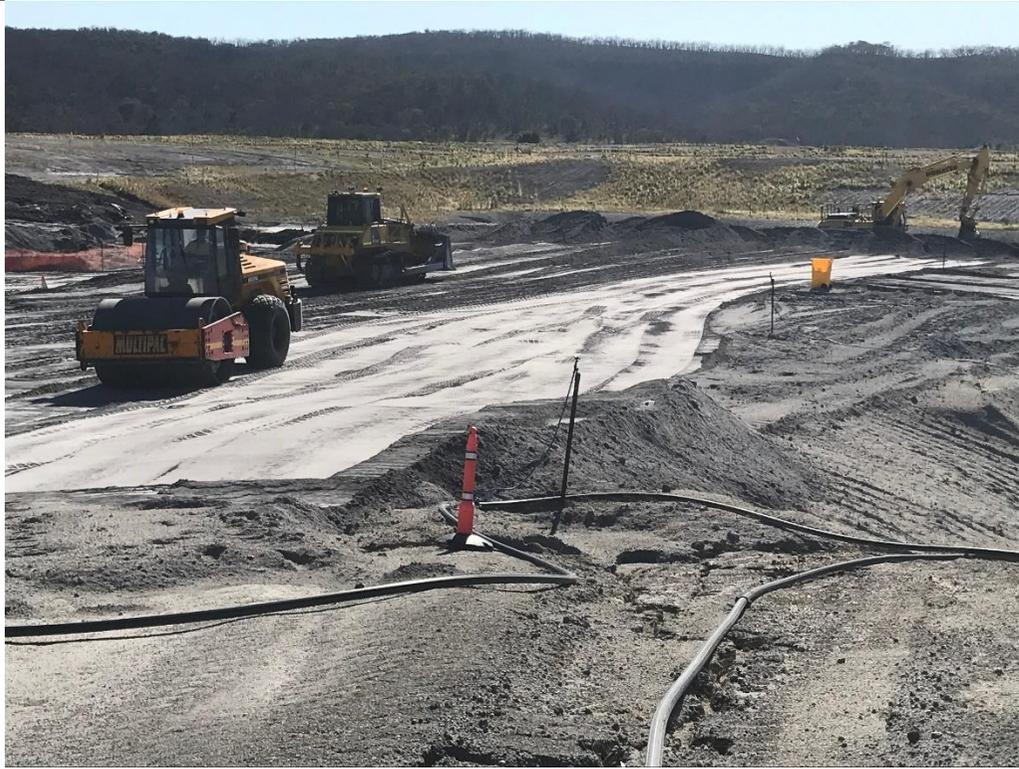
Figure 1 – Compaction activity at Lamberts North Ash Repository (January 2021)
