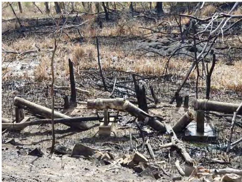
Plate 9: Fire damage to asbestos pipeline, 8 Sept 2020
