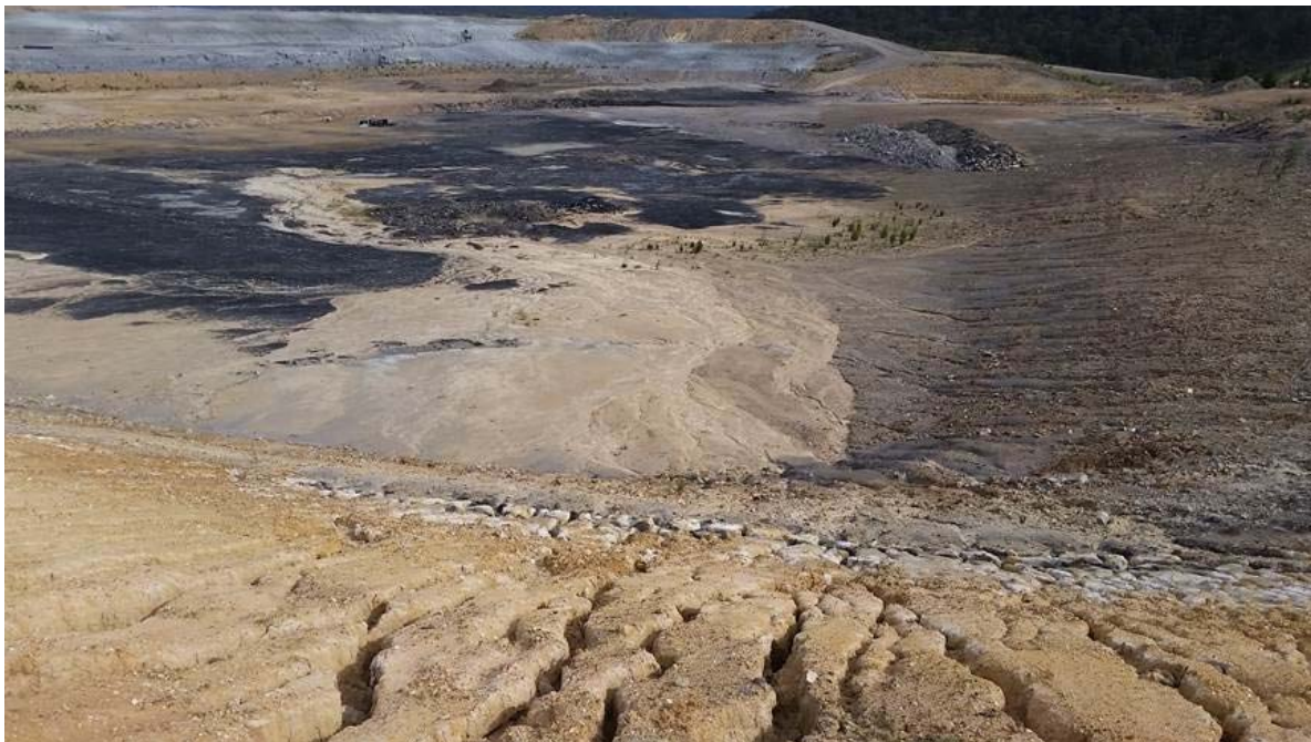
Plate 3: Excavated area of KVAR Stage 2B requires a reinstated soil profile.
