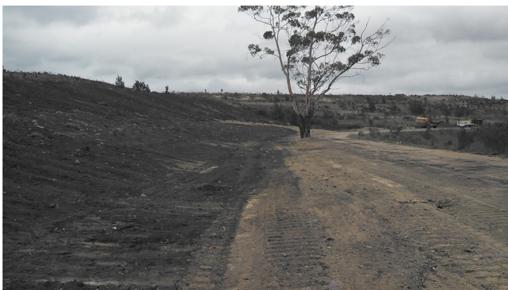
Plate 1: Kerosene Vale Ash Repository Stage 1 rehabilitation earthworks, (batter covered with a green waste compost)
